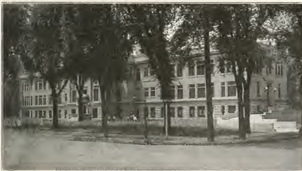
A day school and observation hospital combined in Lymanhurst in Minneapolis
